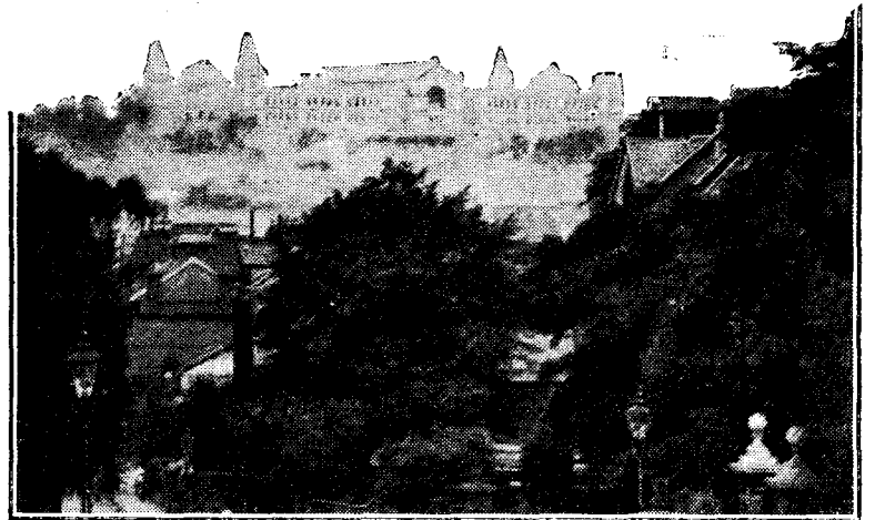
View of the Alexandra Palace, which has been chosen as London's first transmitter site. The top of the south-east tower has been dismantled in preparation for the erection of a transmitting mast.
